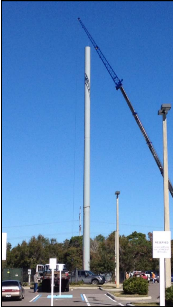
160' Unipole at Gulf Trace ES (Feb 2014)
